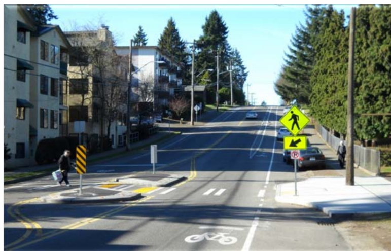
SDOT is already experimenting with standard and buffered bike lanes in uphill locations
